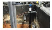
manufacturing of metals, ceramics and other materials, where process temperatures can easily exceed 400 degrees. Here, a LG10 is installed in a waste sump at a metal manufacturing plant. The guided wave sensor is unaffected by the high temperature, condensation and foam.
